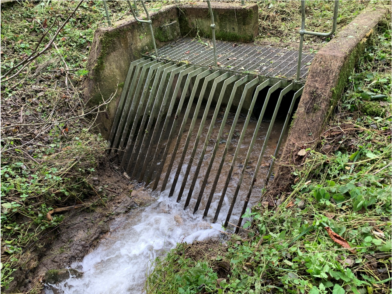
Photograph 3-3 Existing culvert entrance under A417 - tributary of Norman's Brook
